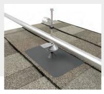
**4.** Drive lag into roof decking until secure.
